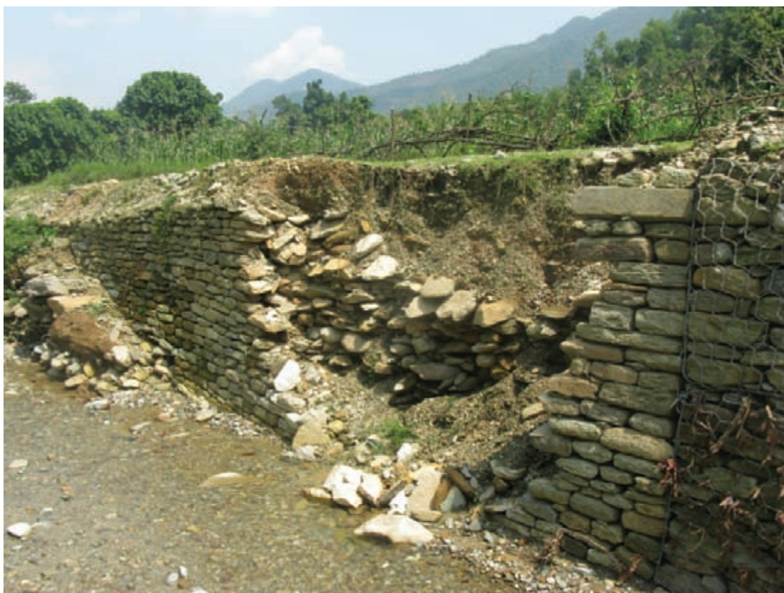
ADB-financed project: defective work on gabion boxes
